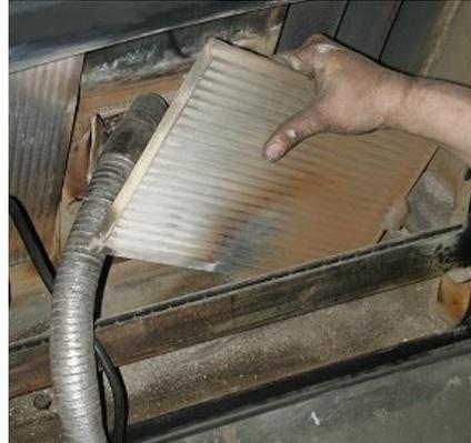
Clean the front and back of the cast iron heat exchanger panels (Fig. 23). Once these cast iron panels are removed, the v-shaped interior accordion heat exchange walls can be cleaned (Fig. 24 & 25).
